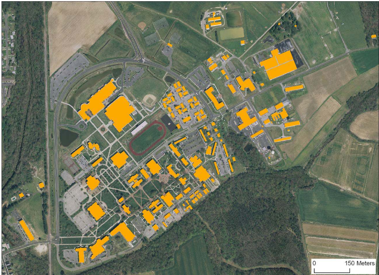
Figure 1 Location of Buildings on UMES Campus
