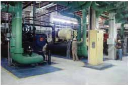
Central Chiller Plant Example
