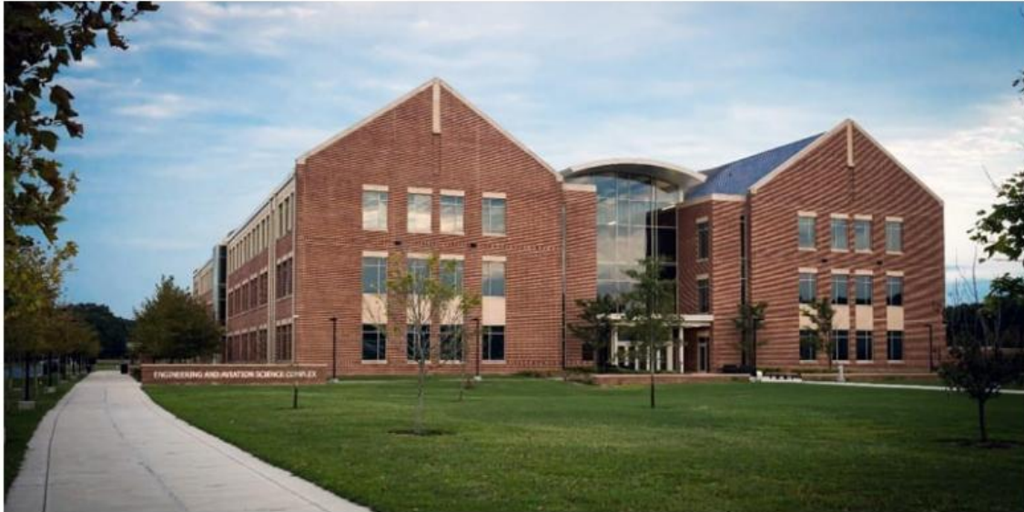
The Engineering and Aviation Science Complex at the University of Maryland Eastern Shore. Image Credit: UMES
